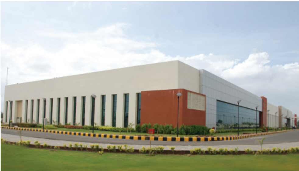
Switchgear Factory, Baroda
