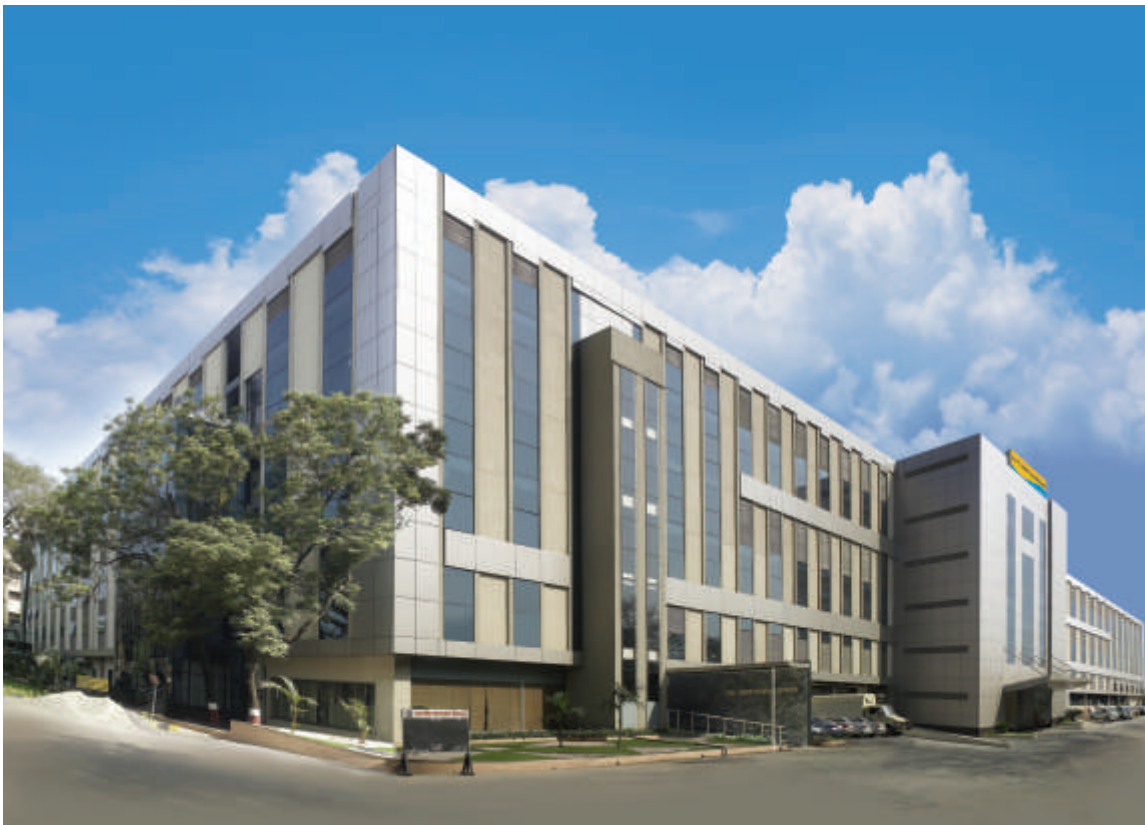
Switchgear Factory, Mumbai
